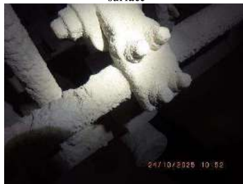
Picture 43: DE hammer was intact
