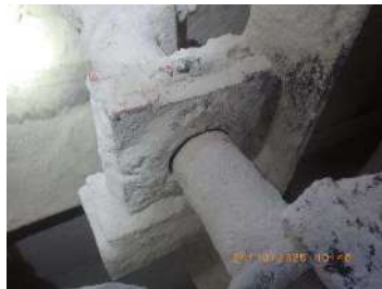
Picture 31: CE bearing still in good condition
