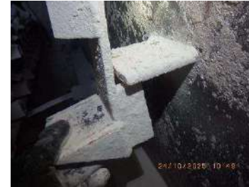
Picture 11: GD anvil still in good condition
