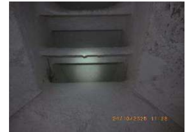
Picture 14: Dust accumulated at outlet
