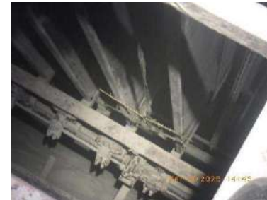
Picture 73 and 74: GD test at top level shown 1.93 m/s
