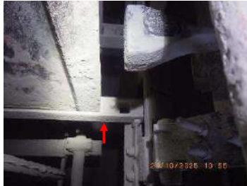
Picture 28: CE bottom bar still in good condition
