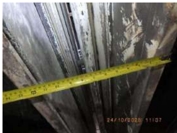
Picture 24: CE – CE gap about 300mm.
