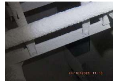
Picture 54: DE bottom bolt was intact
