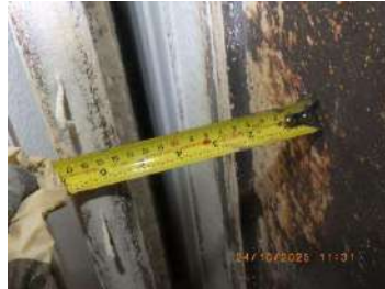
Picture 56: DE - CE gap about 140mm
