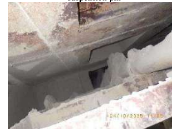
Picture 38: Dust accumulated on DE suspension beam
