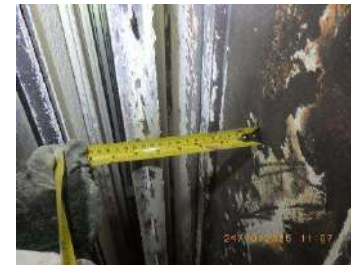
Picture 34: DE – CE gap about 140mm
