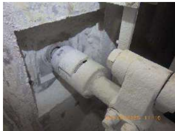
Picture 49: CE coupling was intact
