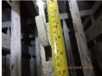
Picture 48: Worn-out CE top hanging
