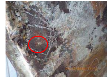
Picture 4: Hole on side access door no. 2
