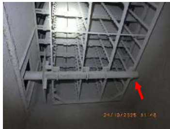
Picture 57 and 58: DE bottom beam seems bending
