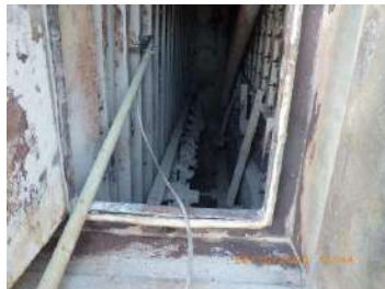
Picture 2: Access door gasket was intact
