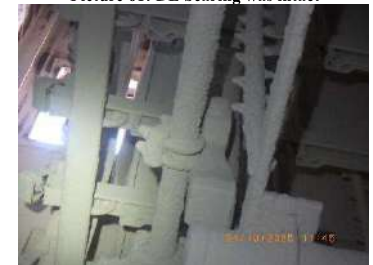
Picture 63: DE hammer was intact
