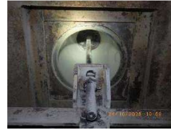
Picture 19: Inner surface of support insulator was cleaned
