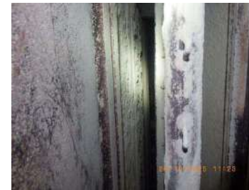
Picture 44: Dust accumulated CE surface at downstream
