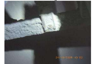
Picture 37: DE bottom bolt was intact
