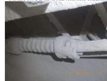
Picture 62: Dust coating on rapping insulator surface
