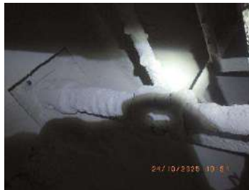
Picture 41: Dust coating on rapping insulator surface
