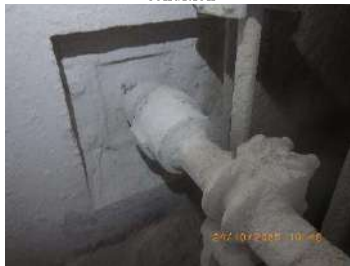
Picture 30: CE coupling was intact
