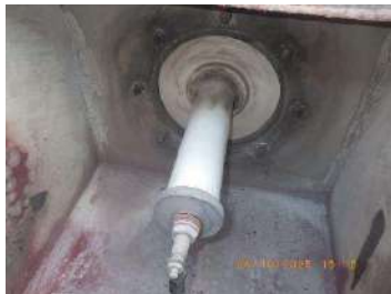
Picture 18: Inside lead-in insulator chamber was cleaned
