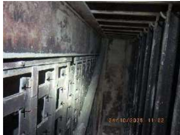
Picture 7 : Intact bolts at the top of GD screen
