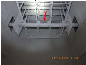
Picture 57 and 58: DE bottom beam seems bending
