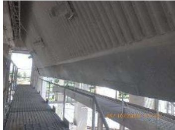
Picture 22: Hopper casing still in good condition
