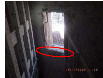
Picture 5: Hole on entry access door no. 3
