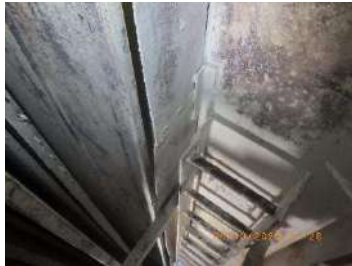
Picture 15: Intact side baffle plate
