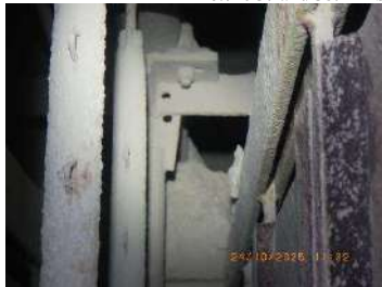
Picture 59: Dust accumulated on DE suspension beam
