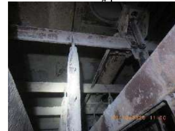
Picture 36: Top DE still connected with suspension pin
