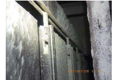
Picture 27: CE top hanging was intact and good condition
